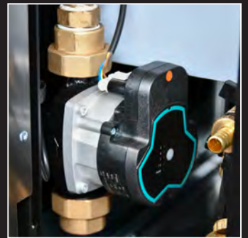
Circuit pump of heating
